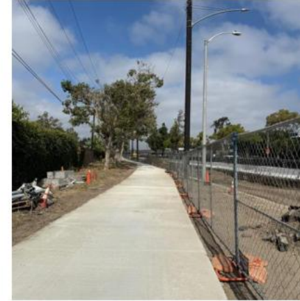
Sidewalk demolition and reconstruction
