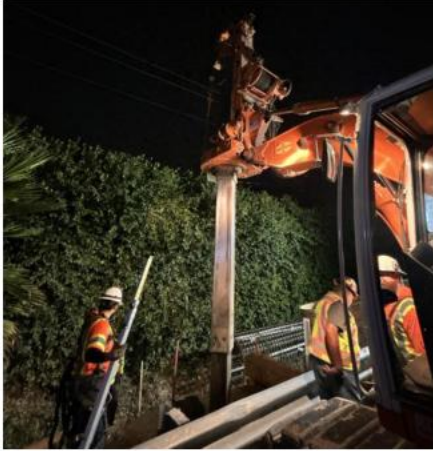
Overhead sign structure excavation
