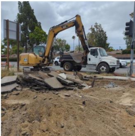
Roadway work: K-rail placement, restriping and roadway excavation
